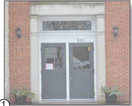
① HOLLOW METAL DOORS & WOOD FRAME
